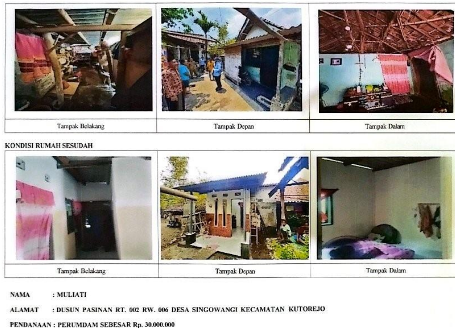
Figure 2. Observation Documentation of House Conditions Before and After Repair (Beneficiary Families) Source: Researchers Documentation (2026)
