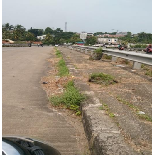
Figure 8. Road Over a Slum Flyover
