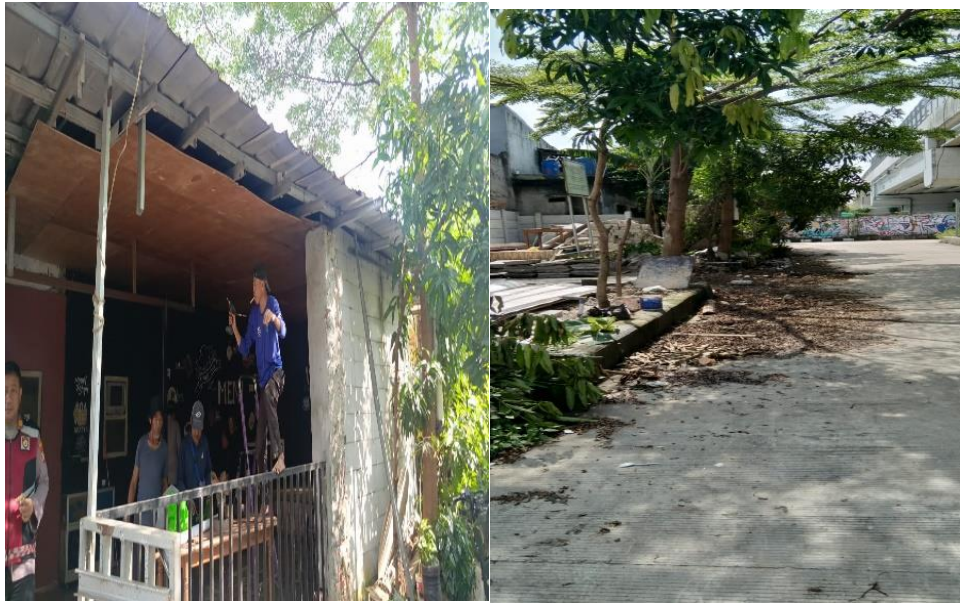
Figure 10. Demolition of Buildings on Toll PU Land
